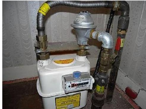
Example of a gas meter with shut of valve located on pipework (red handled lever)
