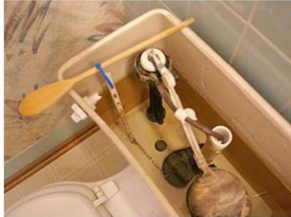
Example of supporting a “Ball Valve” float to stop overflow
